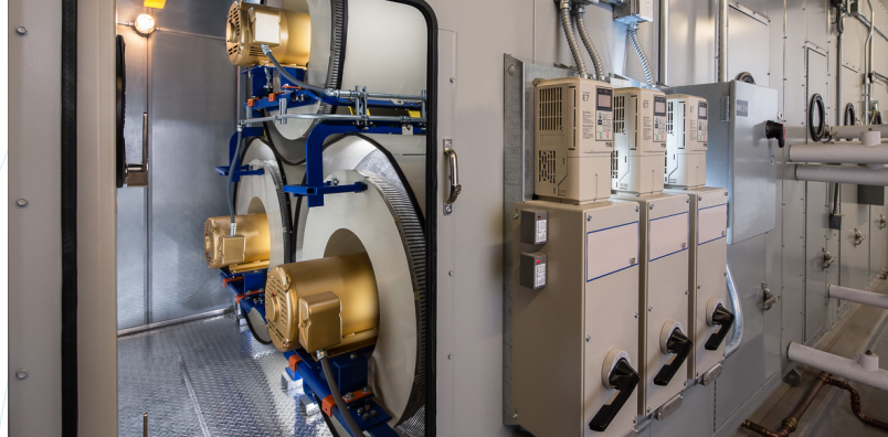
▲ AHU with three AcoustiFLO modules
